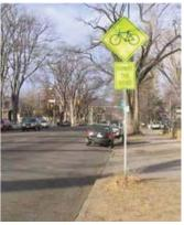
The Manual on Uniform Traffic Control Devices signs in the figures below on urban streets should be installed no less than every 1/2 mile. On rural roads, signs should be installed every 1/4 to 1/2 mile.
